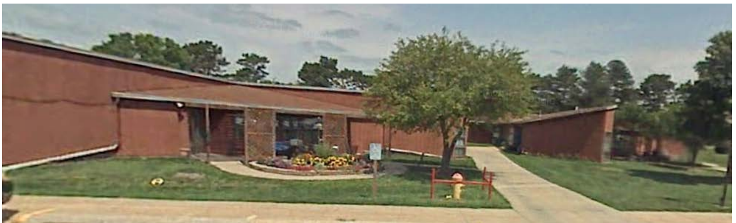
The Solar Cottages had 32 residents at the time of the inspection that found the intermediate living complex deficiency free.
